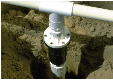
Some drip or solid set installations call for pressure regulators to be installed below ground.
