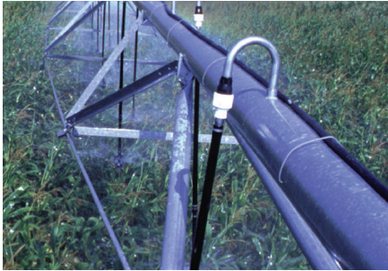
Pivot installations can employ pressure regulators used at the top of the drop pipe or near the spray nozzle.
